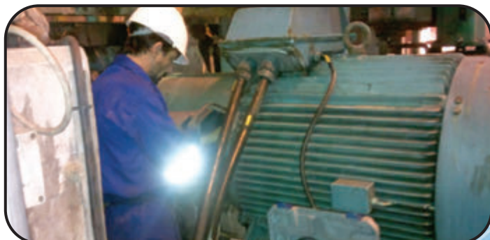
On-site Installations of Earthings at SAPPI SAICCOR
