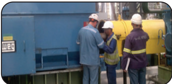
On-site Installations of Earthings at SAFFEL STEEL
