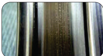
Brown marks from electrical arcing
